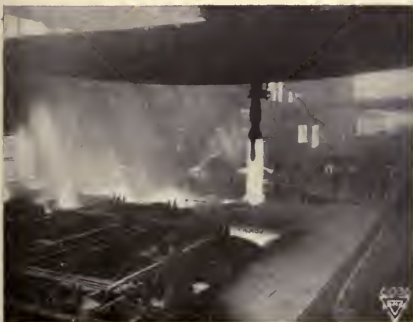
LIFTING HEATED INGOT FROM SOAKING PIT
